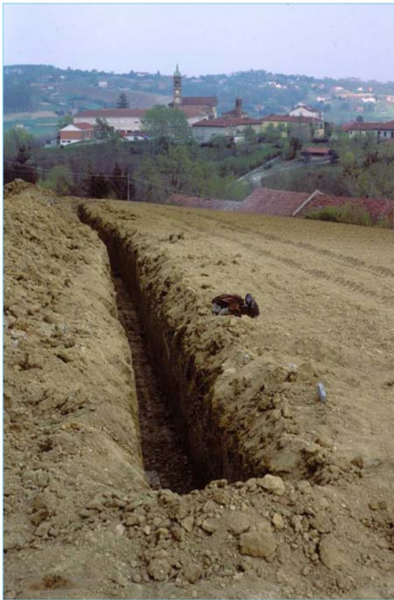
Fig. 15 - The trench located SW of Villafranca d'Asti (the village is located in the background of the photo) cut to study the paleosol between the LC and the UC.
