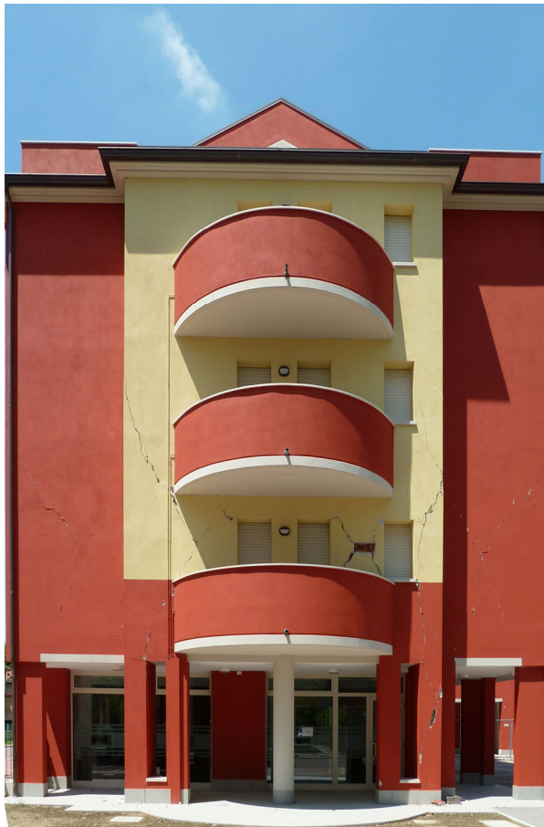
Fig. 13 - Left, Rovereto (Is=I max 7-8 MCS): level 3 damage affecting a r.c. building. Right, Mirandola (Is 7 MCS): partial collapse of the under-roof walls of an unreinforced brick-masonry building of the old-centre (photos of May 29).
