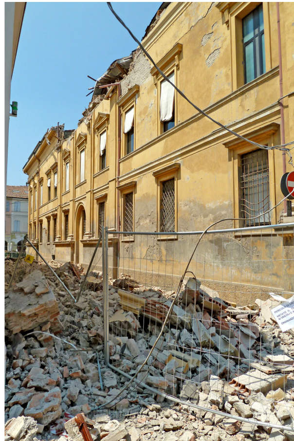
Fig. 13 - Left, Rovereto (Is=I max 7-8 MCS): level 3 damage affecting a r.c. building. Right, Mirandola (Is 7 MCS): partial collapse of the under-roof walls of an unreinforced brick-masonry building of the old-centre (photos of May 29).
