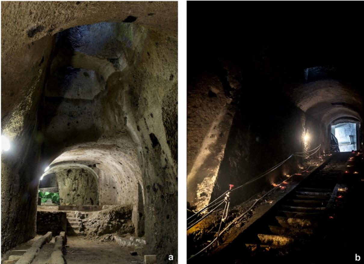
Fig. 3 - Example of cave dug into the tuff. a) view of a chamber with an access well on top; b) details of access realized with steps directly carved into the tuff.
