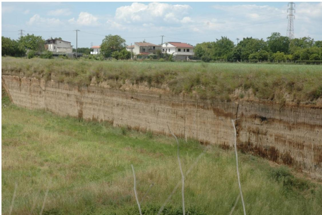
Fig. 4 - A quarry pit showing typical vertical walls, partially filled for agricultural purpose.
