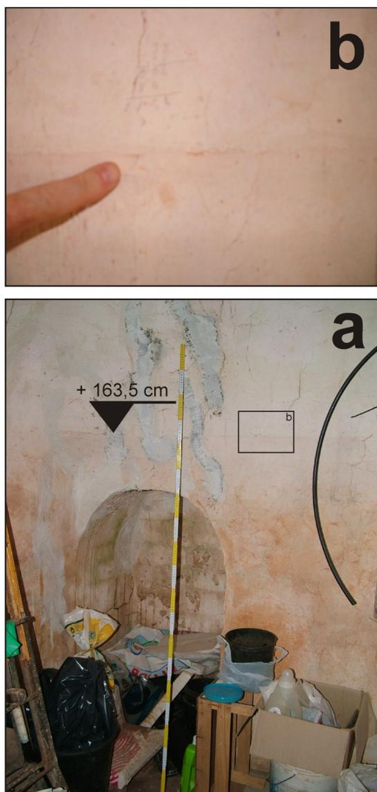
Fig. 9 - Level reached by the 1929 flood detectable by preserved traces on the wall of a historical building (trullo).
