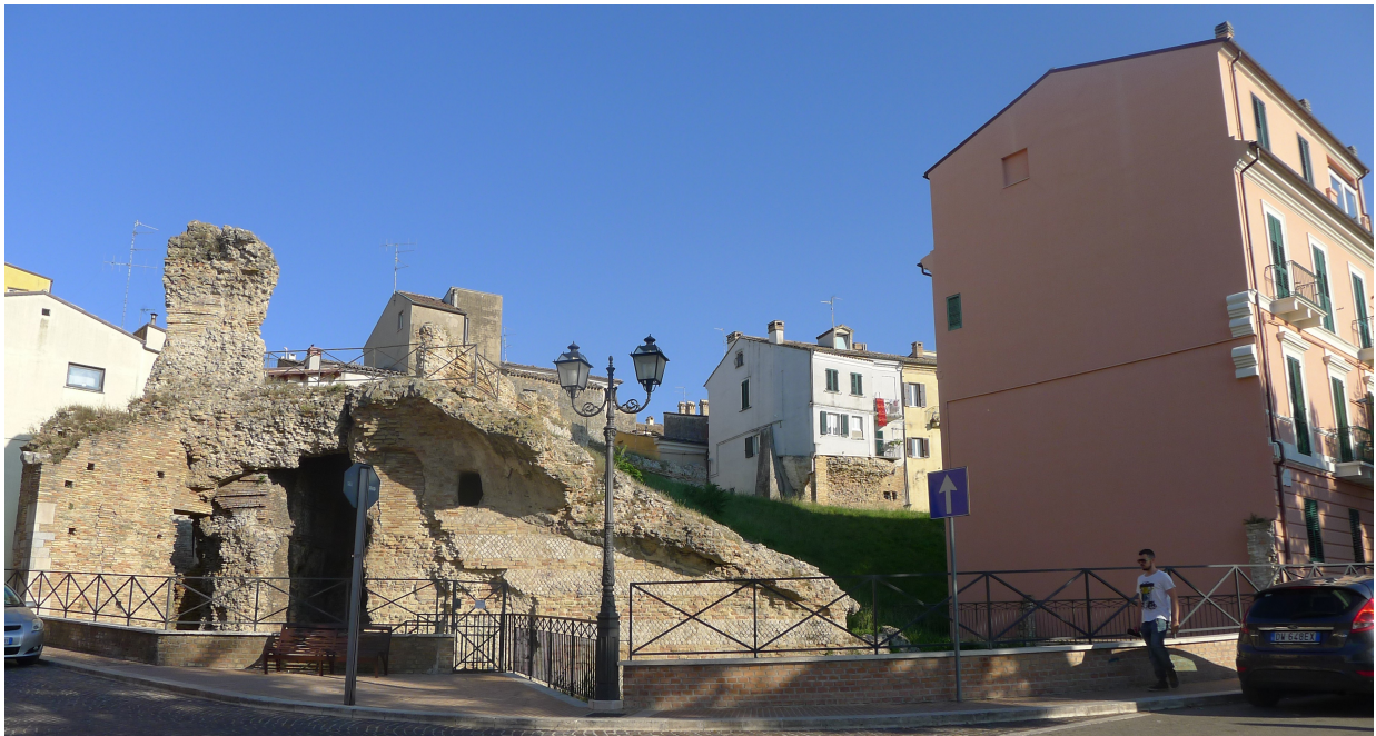
Fig. 7 - The Roman Theater in the upper edge of the western hill slope. The left part of the ring corridor, the Scaenae Frons, the Pulpitum and the Orchestra are missing due to a landslide-associated collapse.
