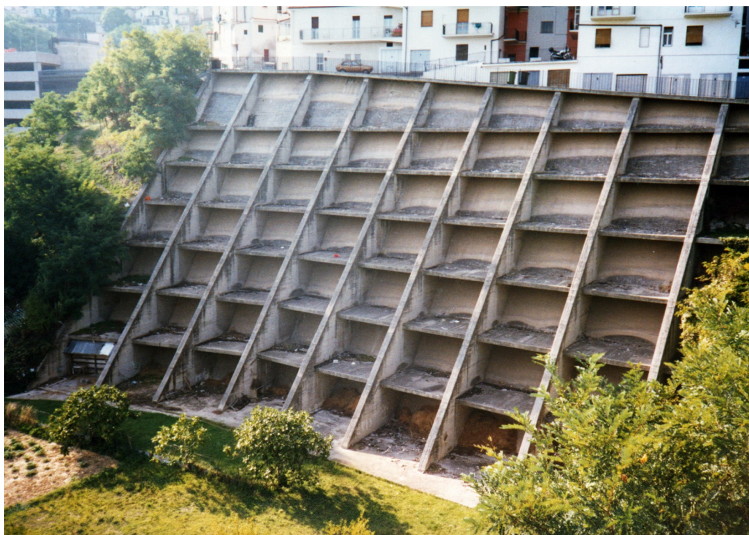
Fig. 9 - Retaining walls on the escarpment edge of the eastern hill slope.
