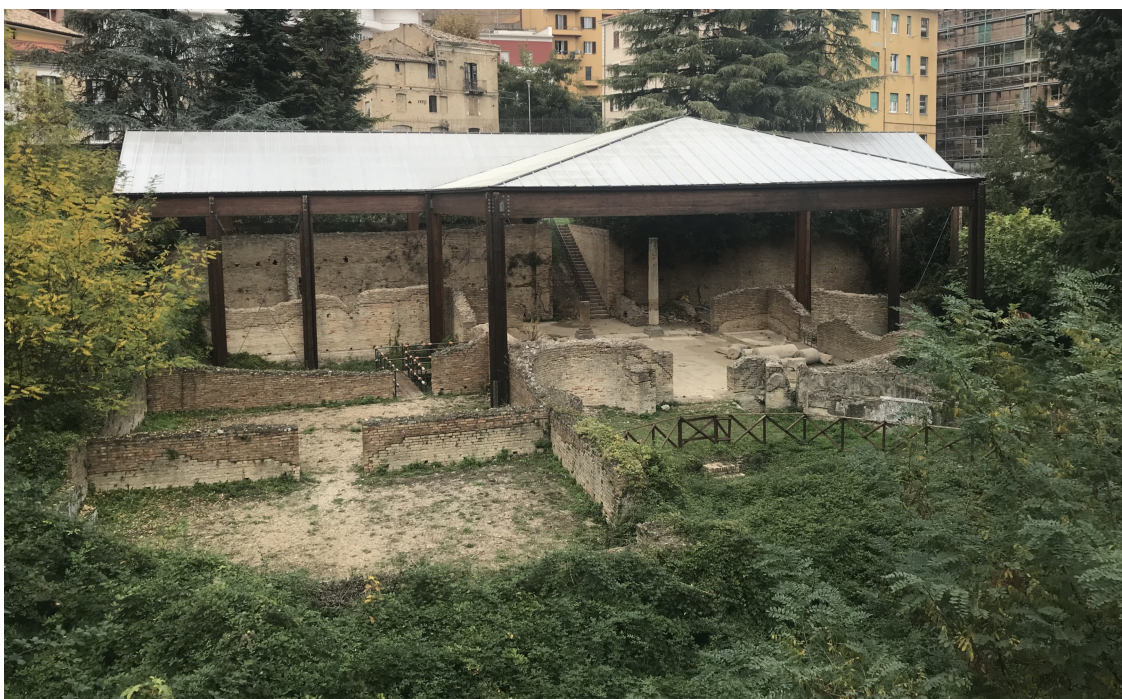
Fig. 10 - Roman Baths and Cisterns area. The right portion of the Roman bath collapsed following a sliding landslide (probably in the 18th century) and recently reconstructed in the 1950s. The 19th century buildings and the road have been build over the cisterns while the urban modern buildings lie over the steep eastern hillslope and the escarpment edge.
