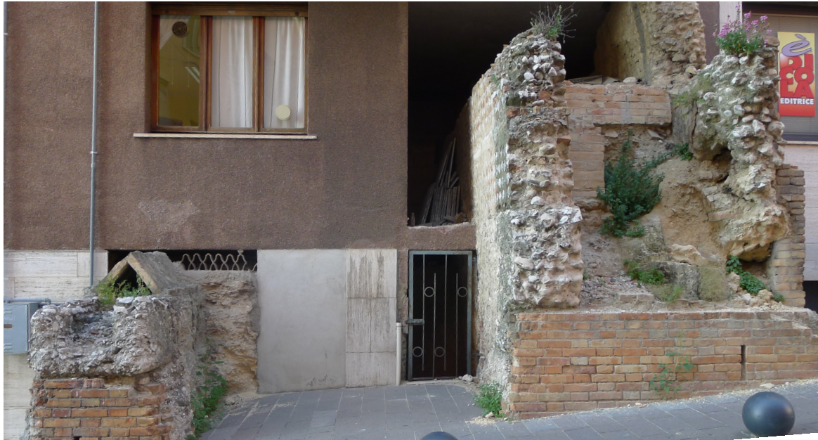
Fig. 8 - Retaining walls and drainage tunnels of the Roman age on the edge of the western hill slope.
