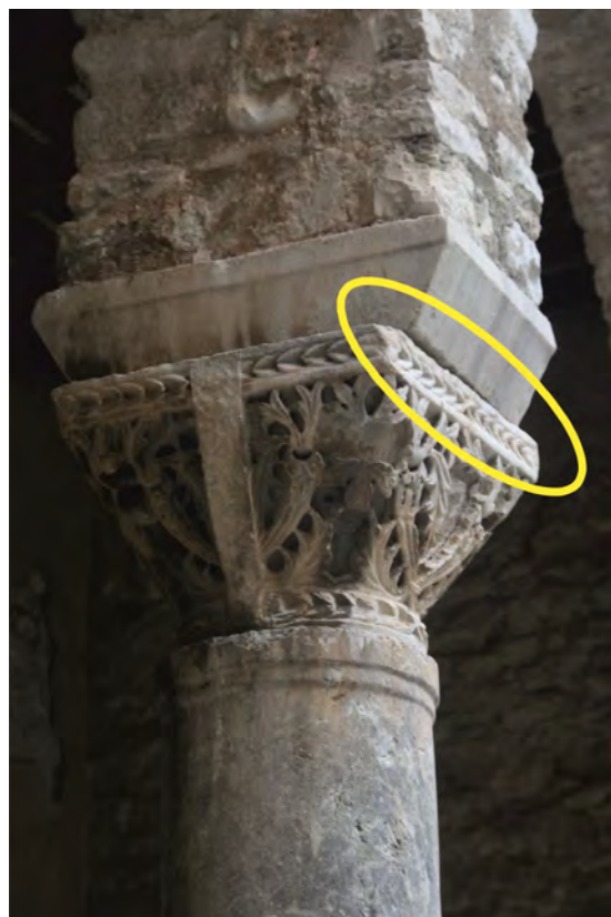
Fig. 4 - Capital of a column in the narthex (forecourt), slightly rotated counterclockwise. The misfit caused by rotation between capital and plinth is encircled. Courtesy of A. Grynaeus.
