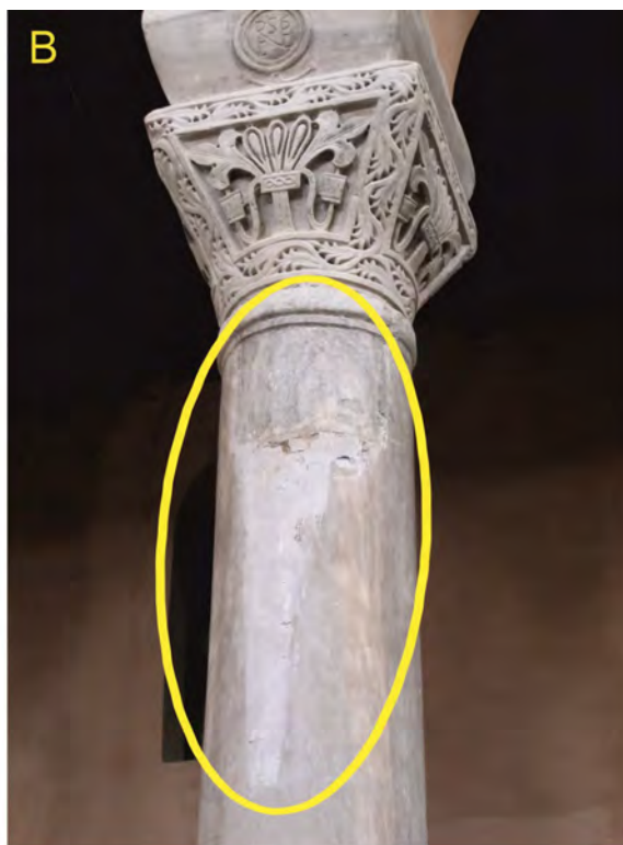
Fig. 5 - Axis-parallel fractures in a marble column. A. Fractures follow schistosity, a zone of weakness. Measure tape extended to 20 cm. ADB photo #2221. B. Fracture not following schistosity. Vertical extent of damage is ca. 1.2 m long. The separated portion of the top 30 cm was reattached during the Medieval restoration, while the remaining portion was replaced with cement. ADB photo #0085.
