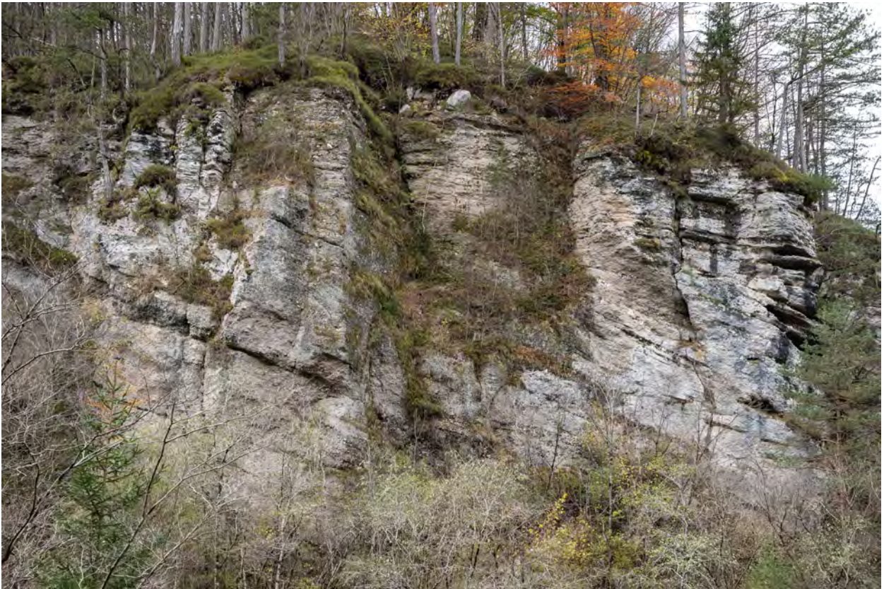
Fig. 9 - Panoramic view of the conglomerate of Gniva (Fig. 1 for position), in the Resia Valley.
