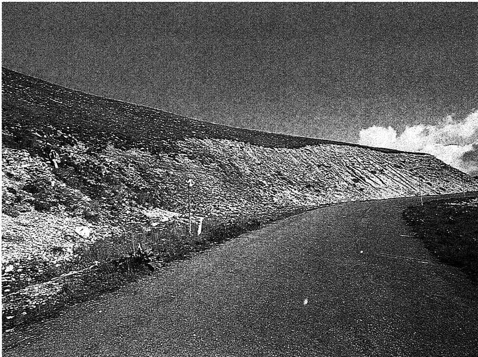
Fig. 16 - The strip of the Valle Cortina ash deposits.
